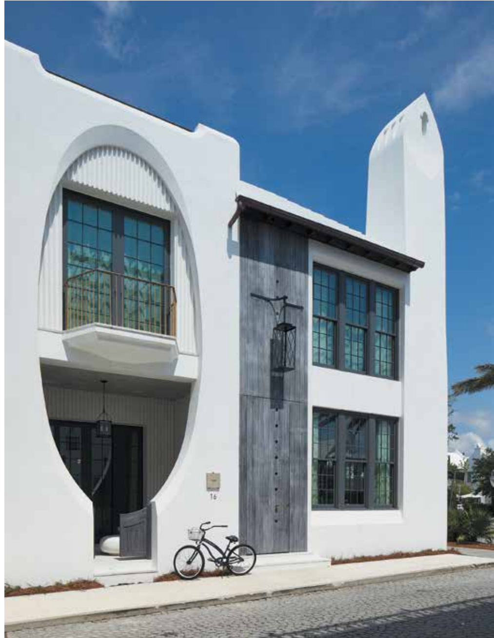
The concrete-and-stucco-clad exterior falls in line with the Alys Beach design direction while standing out from the surrounding structures due to the curvaceous and modern concrete details. OPPOSITE PAGE: In the living room, designer Ohara Davies-Gaetano installed a chandelier from Lucca Antiques, a sofa covered in Lee Industries fabric and a coffee table from Clubcu.
